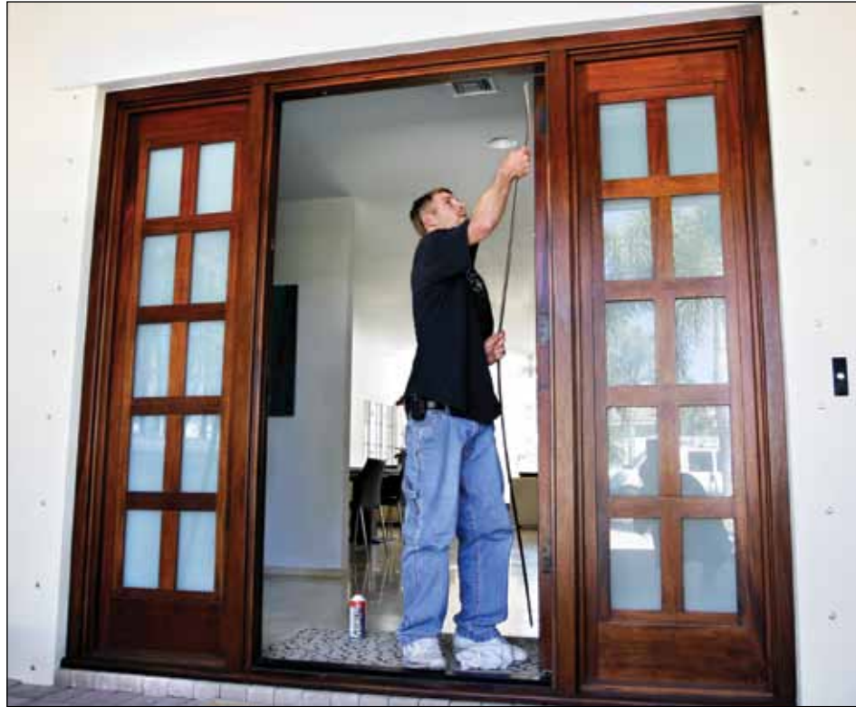
Caretaker Jerred Lockwood adjusts the weather stripping on the front door to a home.
