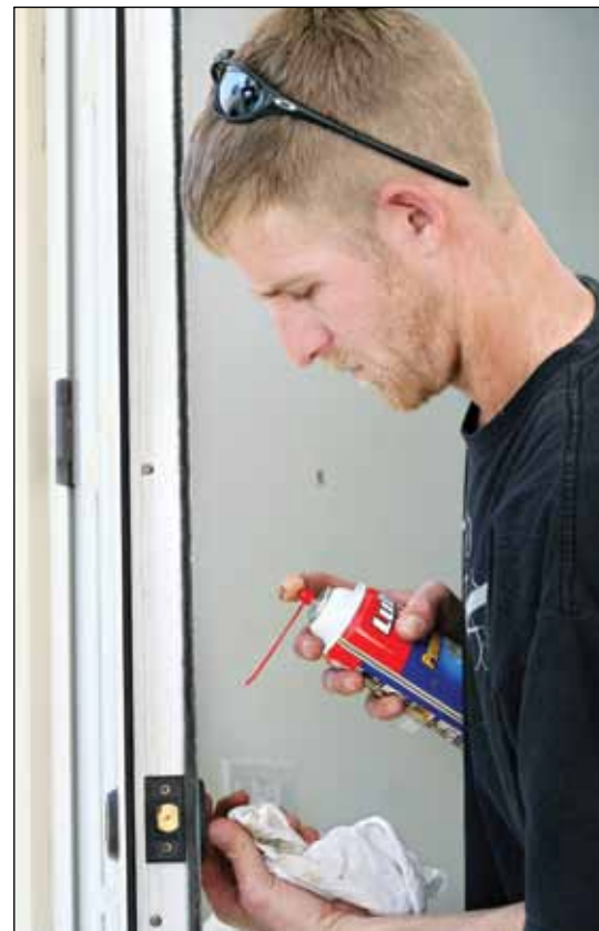
Jerred Lockwood lubricates the locks and hinges on a door.
